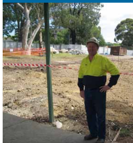
Paul Gilbert on site at Engadine Public School.
