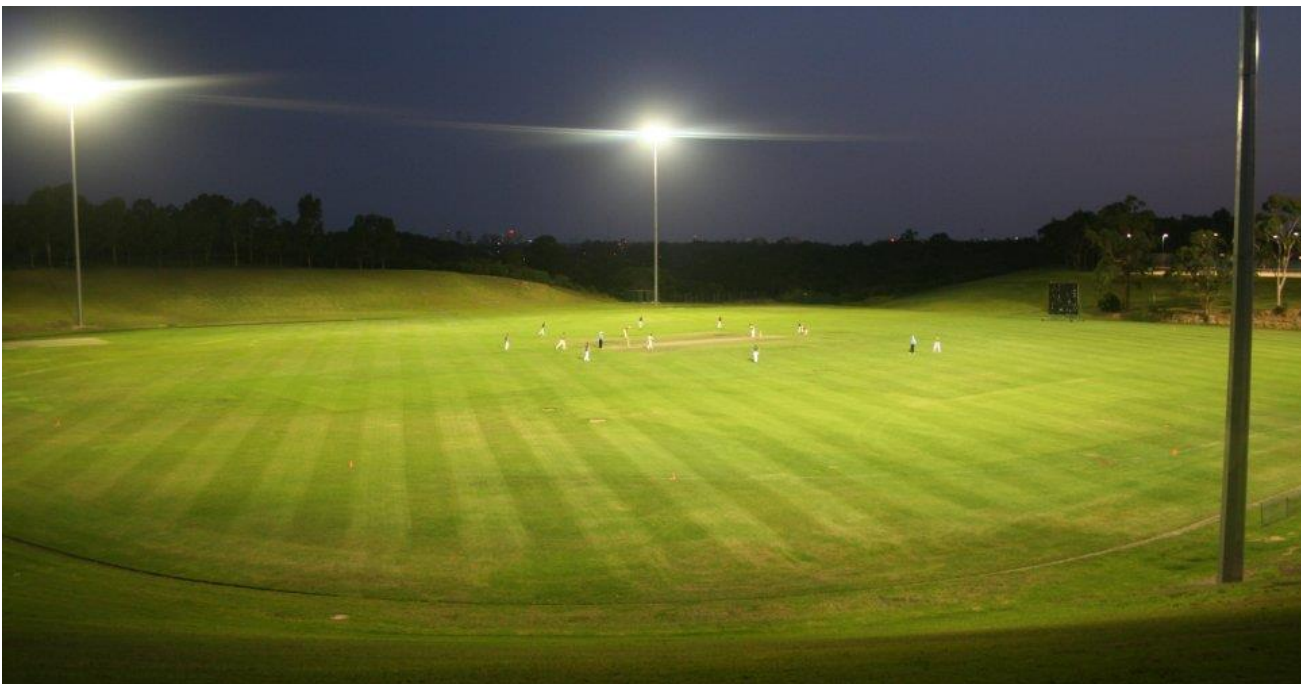
Figure 3-1: Example of A Sports Field in NSW with Four Light Towers Setup
