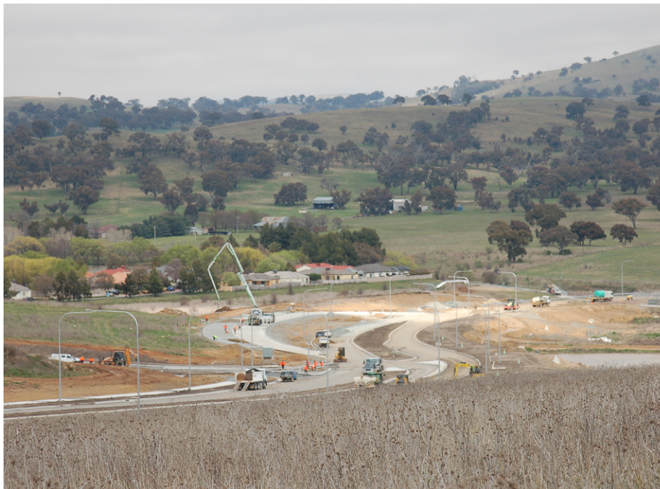
View of the new access road looking south
