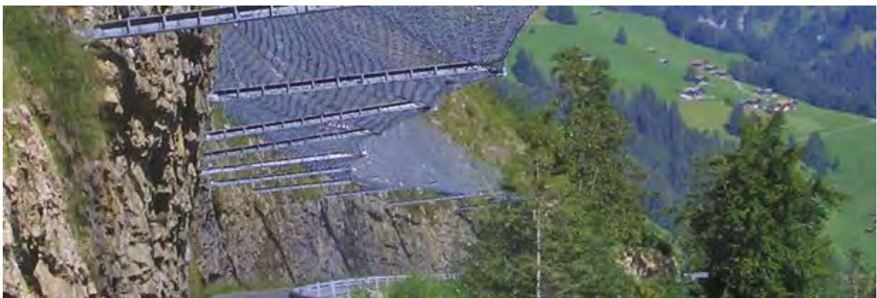
Figure 2 – Example of Rockfall Protection Structure
