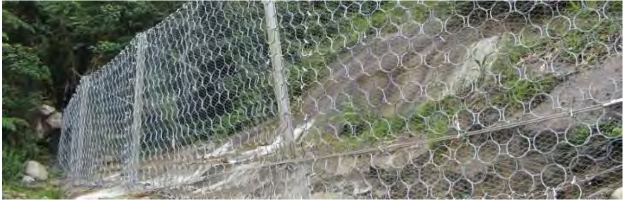
Figure 1 – Example of Rockroll Protection Structure
