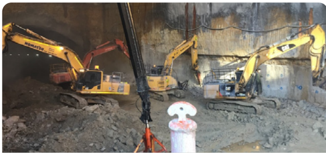
Works on the Sydney Metro
