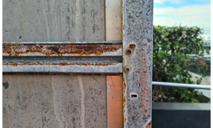
Figure 7: Care must be taken with products formed from galvanized sheet to prevent corrosion
