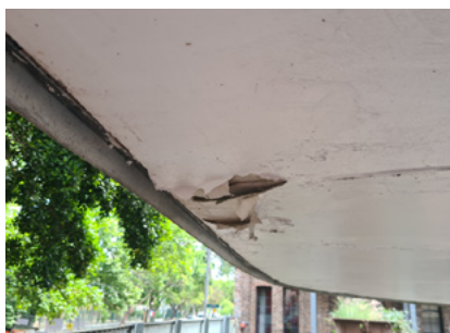
Figure 38: Inadequate weatherproofing resulting in moisture ingress
