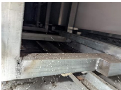
Figure 37: Inadequate fixings of subframing to supporting structure
