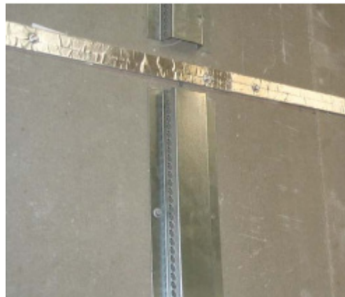
Figure 19: Cavity barriers are to be continuous
