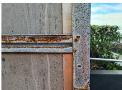
Figure 36: Standard galvanized coatings showing significant deterioration (located within close proximity to the coastline)
