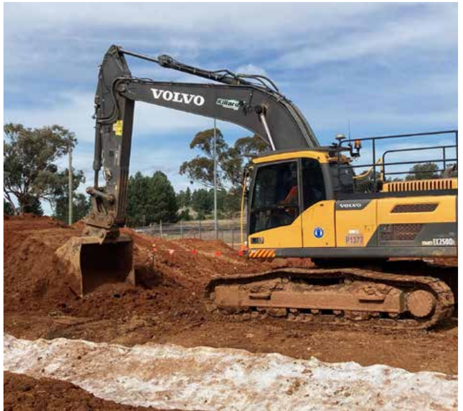
An excavator works on the Parkes precinct enabling works
