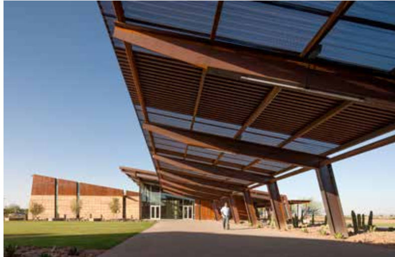
Central Arizona College, USA Cantilevered walkway (sunshading) connecting buildings Courtesy of Bill Timmerman
