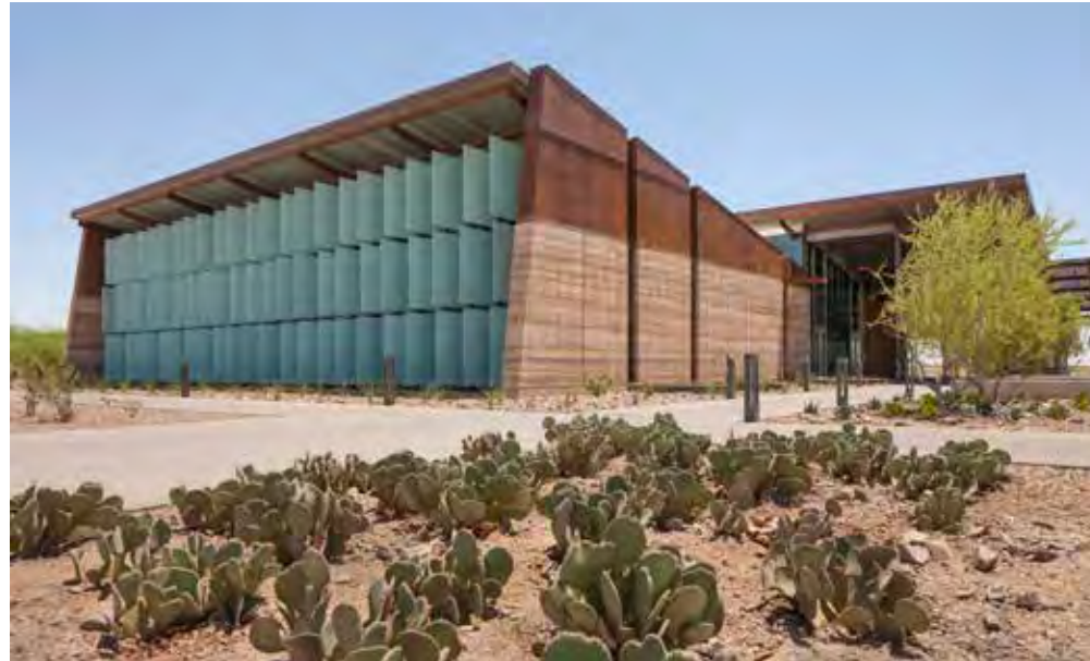
Central Arizona College, Maricopa Use of passive solar shading integrated into the building design
