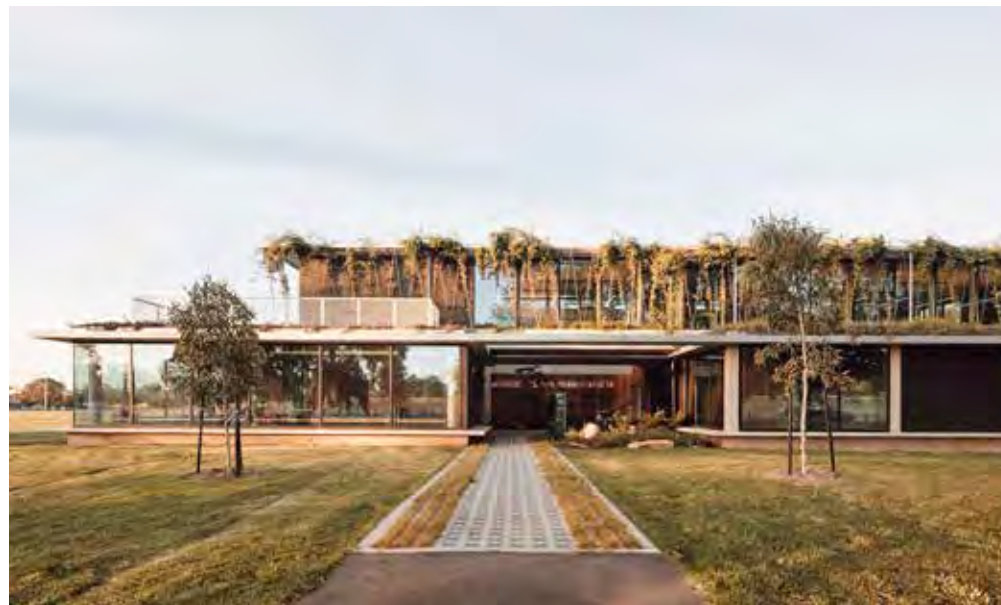
Parks Victoria Depot, VIC Use of laminated timber, greening of building
