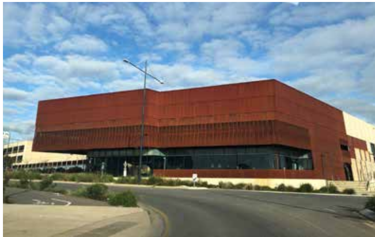
Drill Core Reference Library, Tonsley, SA 'Cor-ten' steel panels and precast concrete
