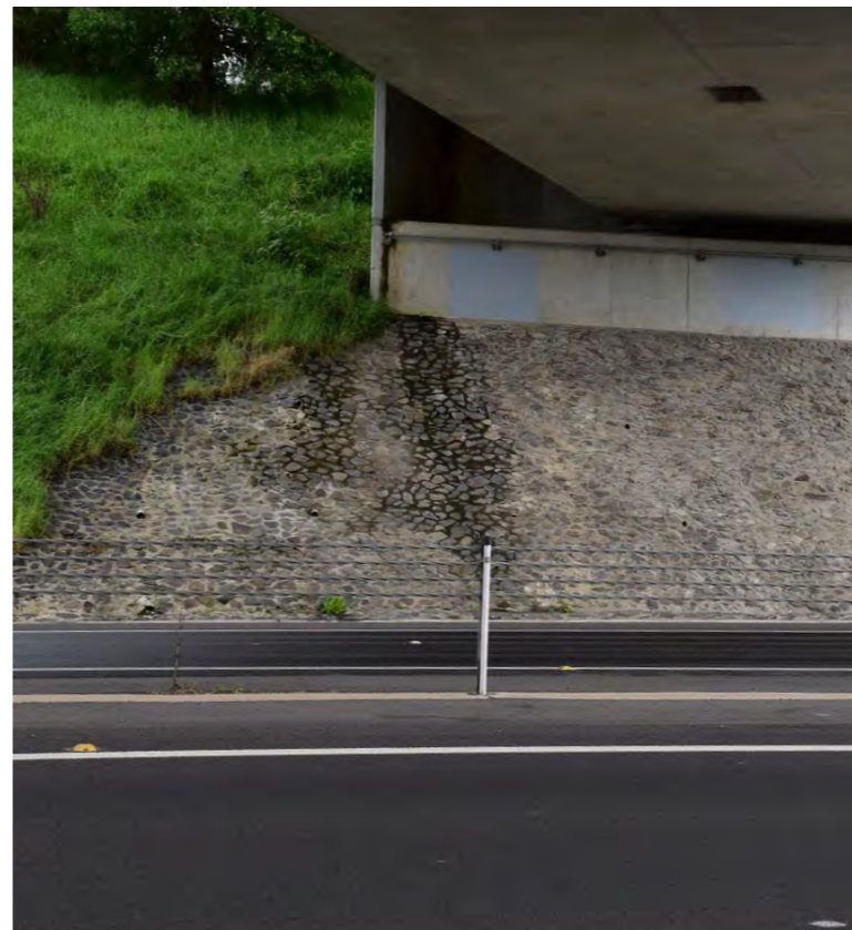
Figure 34. Abutment treatment option 1: stone pitching
