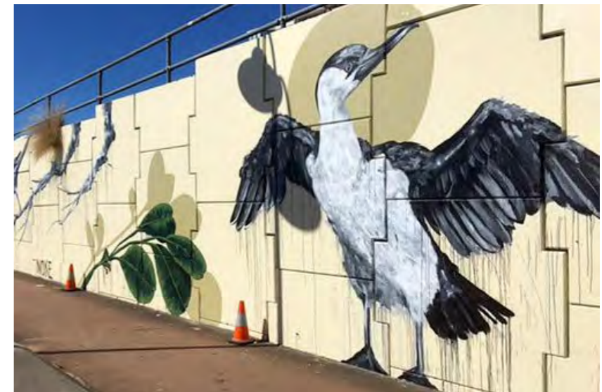
Figure 44. The Birds' mural over plain concrete RSW panels in Dock Street, Brisbane by artist Noke
