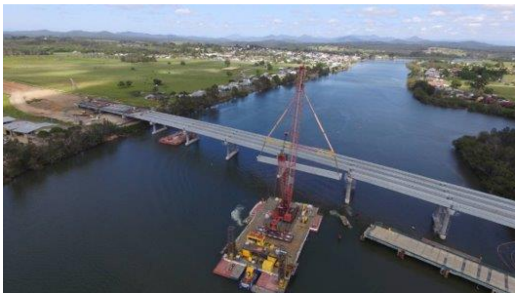
Figure 1: The new Nambucca River Bridge under construction. Photo credit: Macleay Argus.
