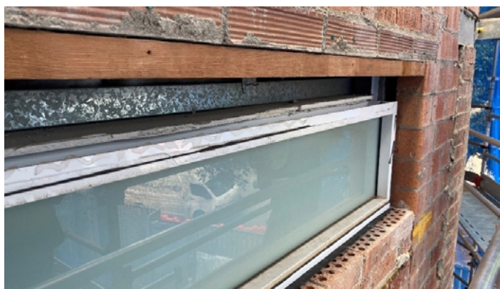
Figure 18.6: Timber lintels
