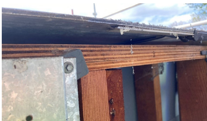
Figure 18.7: Timber parapet framing
