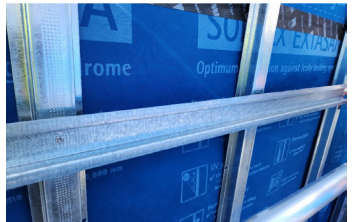
Figure 18.3: Sarking complete with top hat subframe
