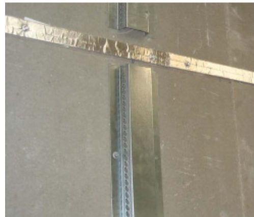
Figure 10.6: Cavity barriers are to be continuous
