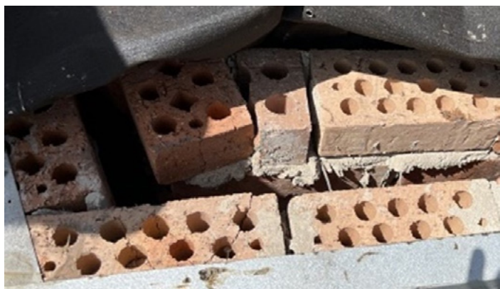
Figure 18.5: Defective masonry construction
