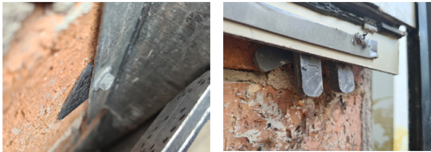
Figure 15.8: Combustible components (packers)
