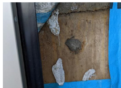
Figure 15.5: Inadequate weatherproofing resulting in moisture ingress
