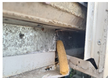
Figure 15.4: Inadequate fixings of subframing to supporting structure
