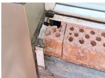
Figure 15.6: Inadequate wall structure
