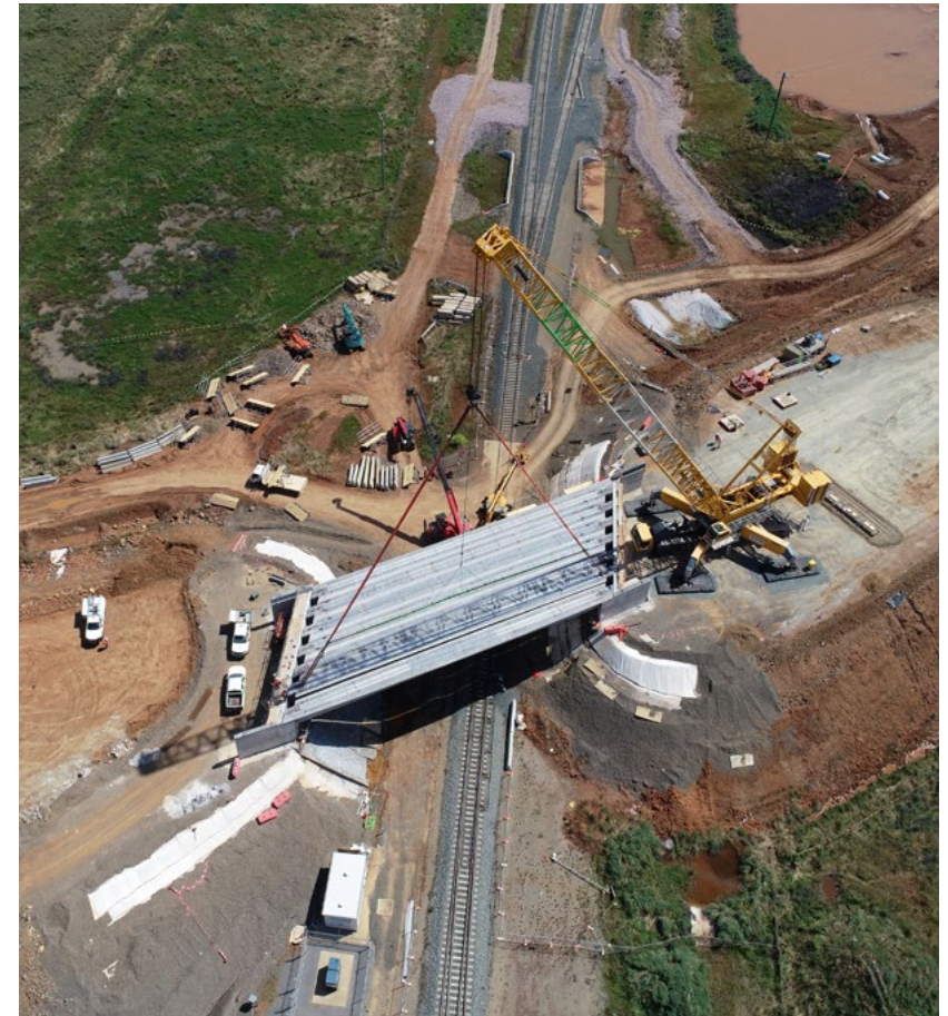
Aerial view of Brolgan Road bridge construction
