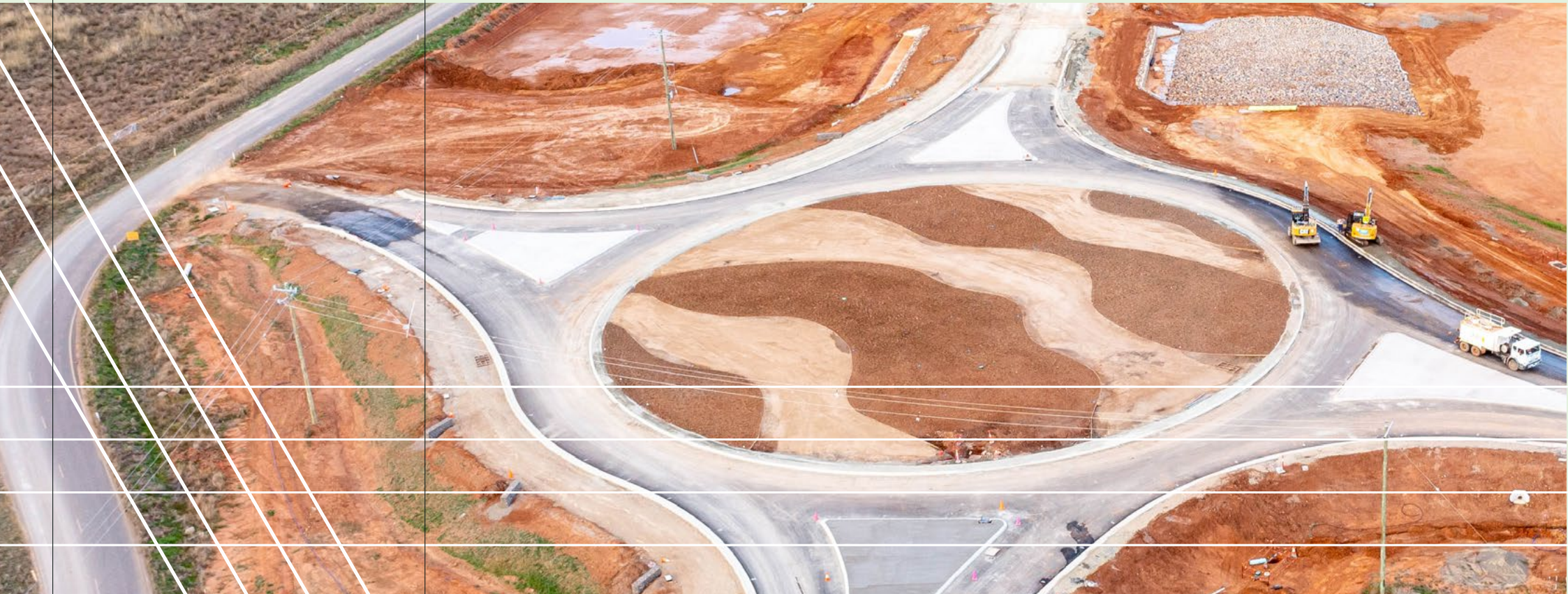
Aerial view of roundabout construction in Parkes
