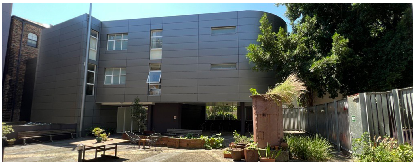
Figure 18.13: View of building (post-remediation works)
