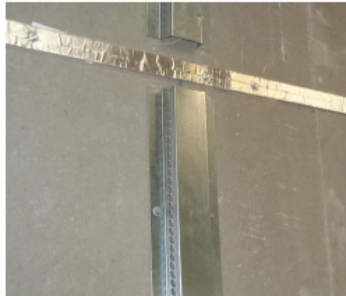
Figure 10.6: Cavity barriers are to be continuous
