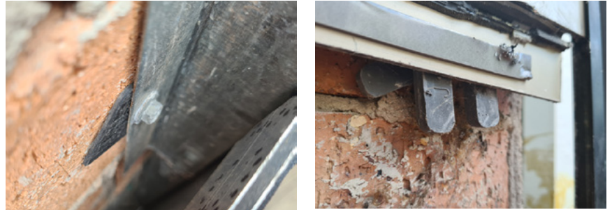
Figure 15.8: Combustible components (packers)
