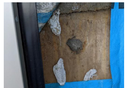
Figure 15.5: Inadequate weatherproofing resulting in moisture ingress
