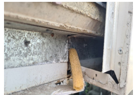
Figure 15.4: Inadequate fixings of subframing to supporting structure
