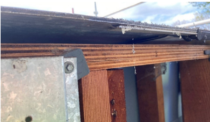
Figure 18.7: Timber parapet framing
