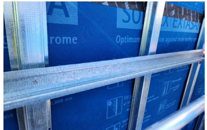
Figure 18.3: Sarking complete with top hat subframe
