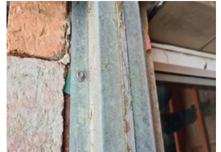
Figure 15.2: Cladding fixed to the supporting top hats with double-sided tape
