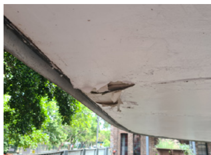
Figure 15.5: Inadequate weatherproofing resulting in moisture ingress
