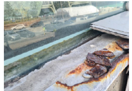
Figure 15.3: Standard galvanized coatings showing significant deterioration (located within close proximity to the coastline)
