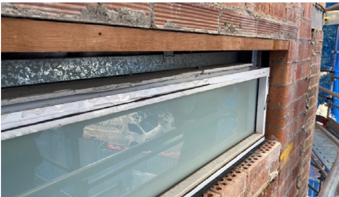
Figure 18.6: Timber lintels
