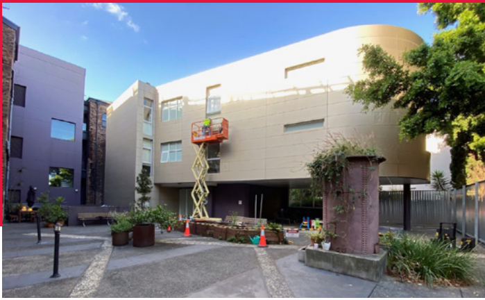
Figure 18.1: View of building (pre-construction)
