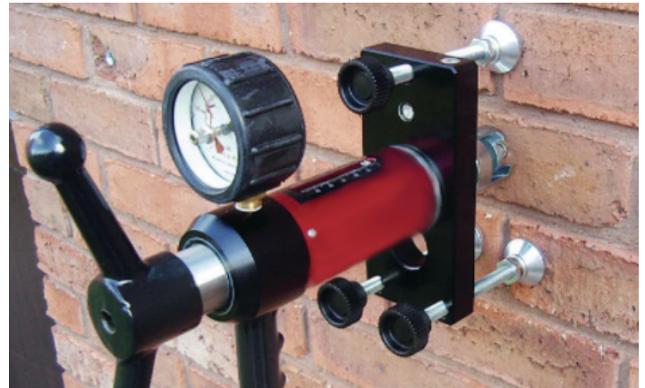
Figure 5.6: Masonry pull-out test
