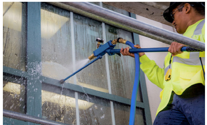
Figure 5.7: Window hose testing
