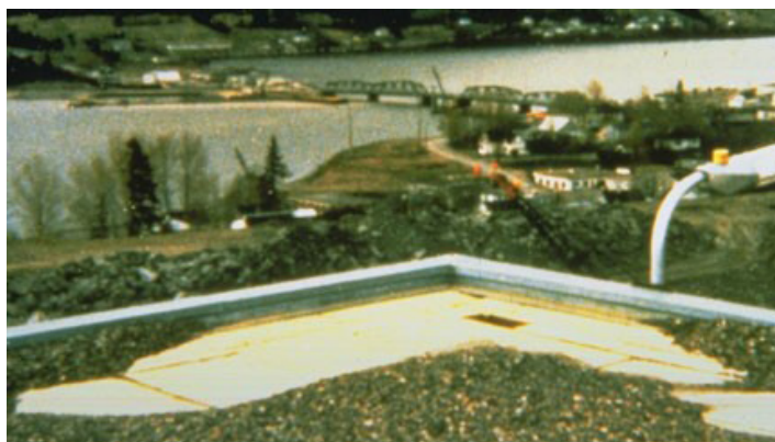
Figure 14.9: Gravel dislodgement to elevated roof due to the two horizontal roof-corner vortices generated by the cornering flow approaching the image (after ASCE Webinars 2005-2012)
