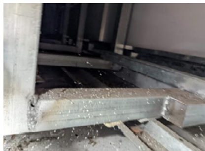
Figure 15.4: Inadequate fixings of subframing to supporting structure
