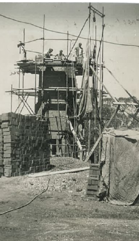
Crookwell Hospital chimney taking shape - 1952.
