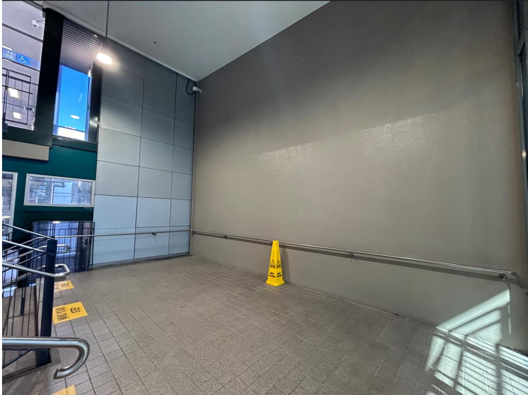
West Stairs (Photo #1)
