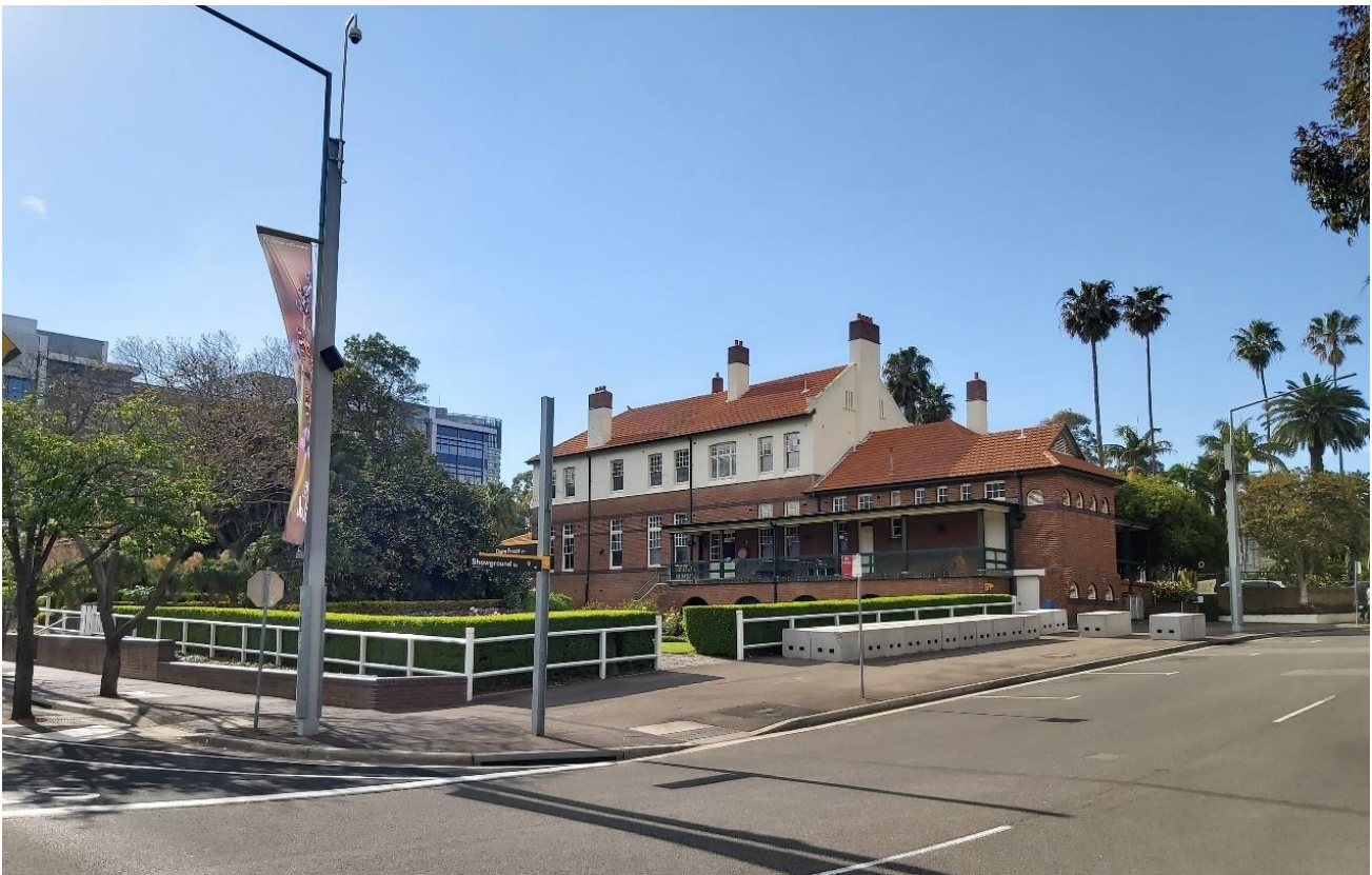
Figure 12.6 View of Federation era building within the State Abattoir locality
