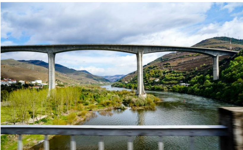
Figure 5.12 Example of box girder bridge
