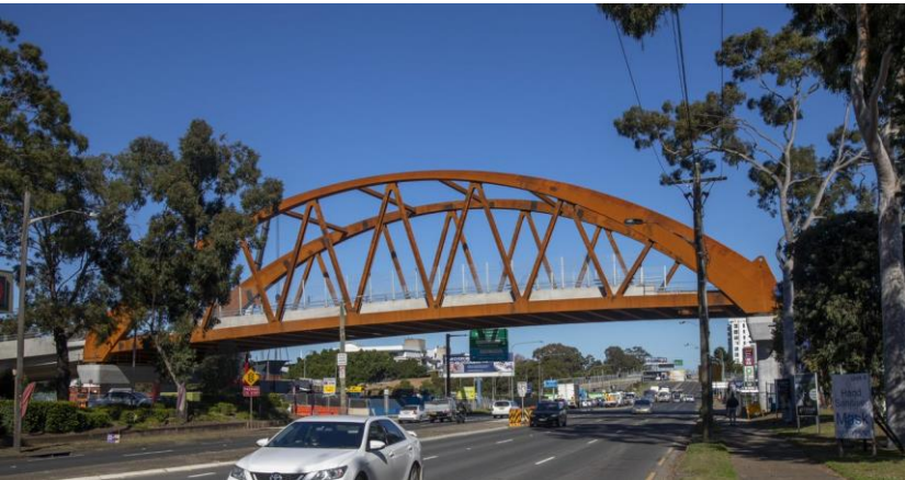
Figure 5.14 Example of a tied-arch bridge
