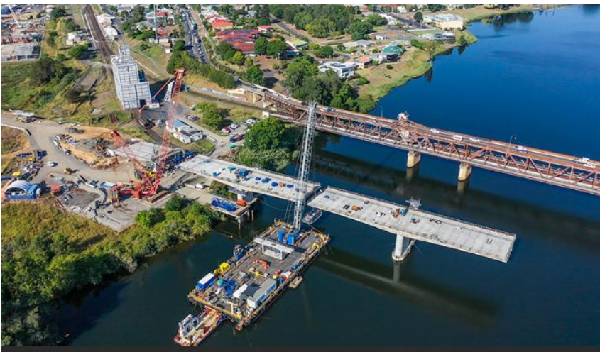
Figure 5.22 Example of bridge construction using a barge
