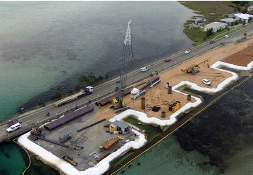
Figure 5.23 Example of bridge construction using a causeway
