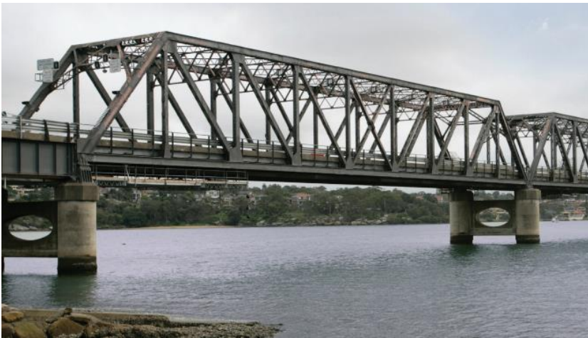
Figure 5.20 Example of a steel truss bridge
