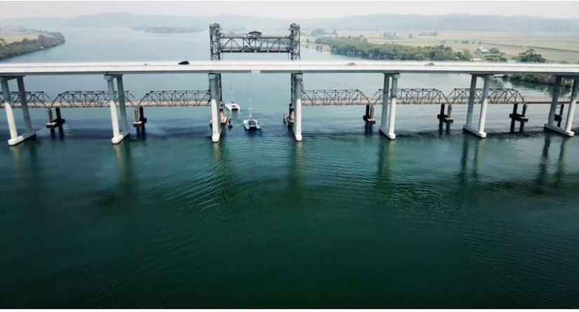
Figure 5.13 Example of a super-T bridge
