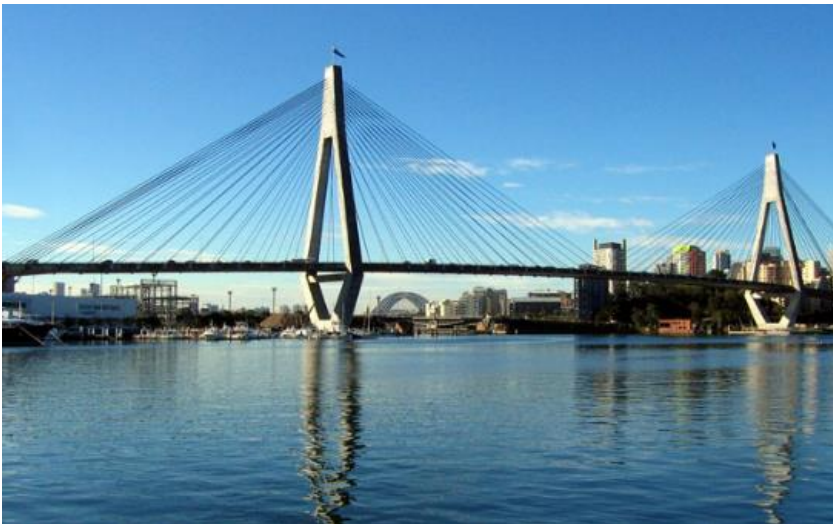
Figure 5.21 Example of a cable-stayed bridge
