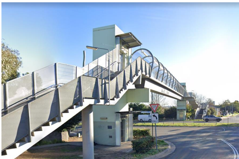
Figure 5.15 Existing pedestrian bridge over Silverwater Road
