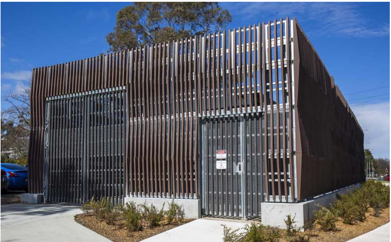
Figure 6.18 Example of traction power substation
