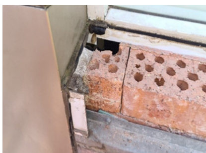
Figure 39: Inadequate wall structure
