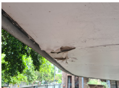
Figure 38: Inadequate weatherproofing resulting in moisture ingress
