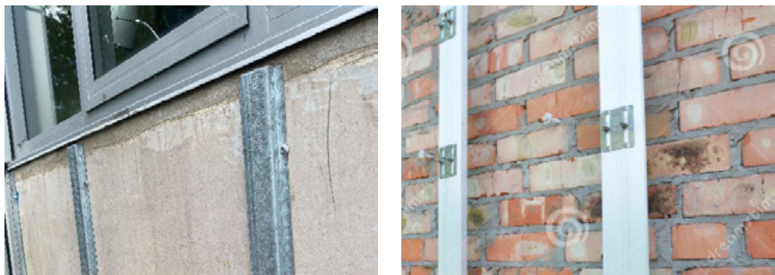
Figure 42: Inadequate or lack of insulation
