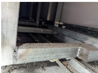
Figure 37: Inadequate fixings of subframing to supporting structure
