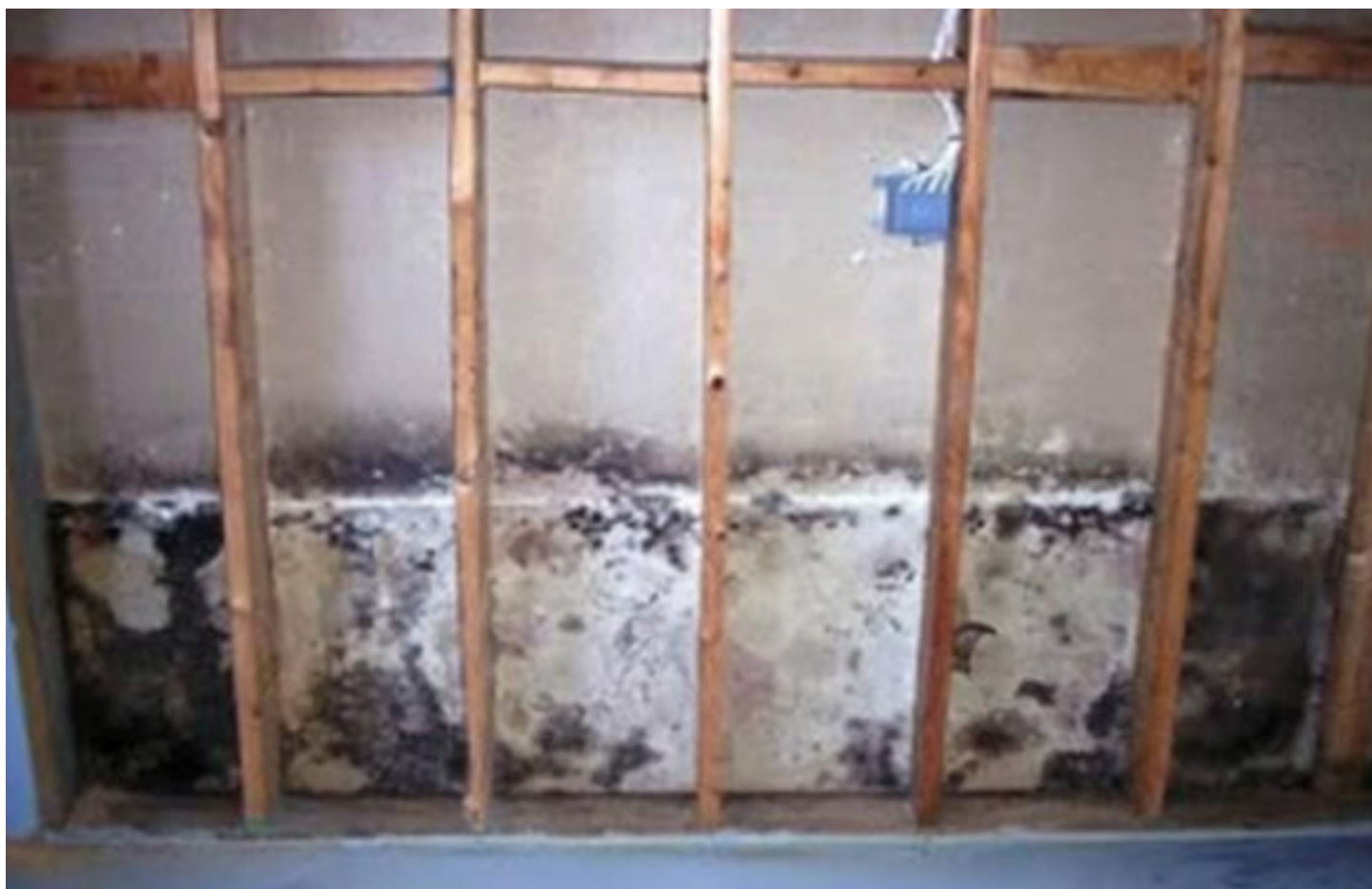
Figure 20: Black mould growth in a wall cavity due to poor ventilation and condensation on inside face of cladding
