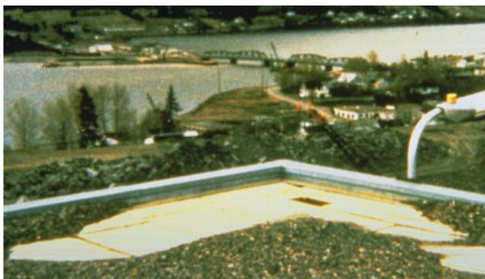
Figure 33: Gravel dislodgement to elevated roof due to the two horizontal roof-corner vortices generated by the cornering flow approaching the image (after ASCE Webinars 2005-2012)
