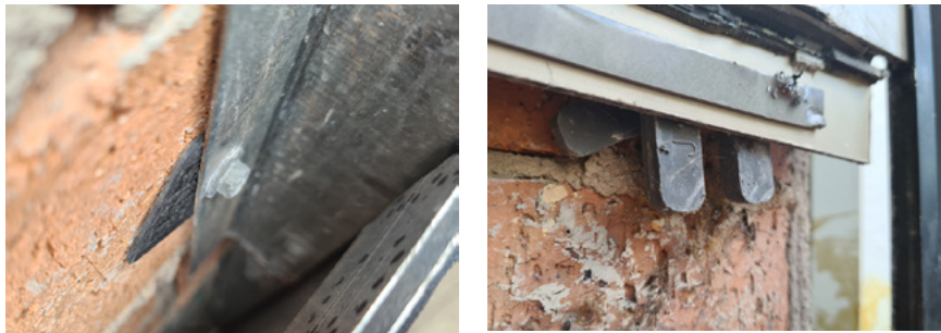
Figure 41: Combustible components (packers)
