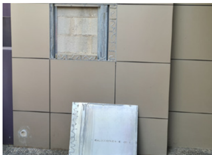
Figure 34: Cladding fixed to the supporting top hats with silicone sealant
