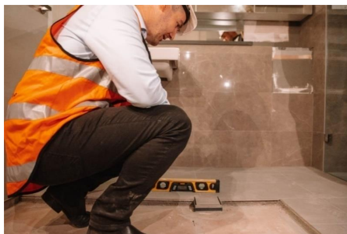
Checking the degree of 'fall' in bathroom tiling
