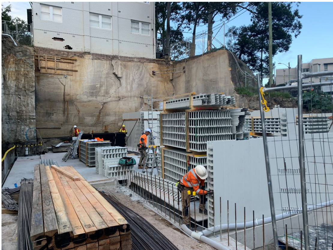
Construction workers on site
