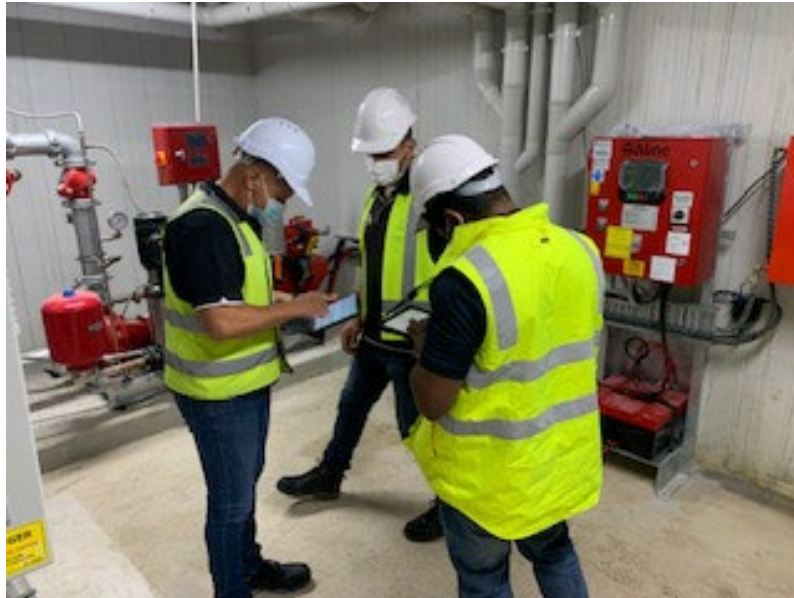
Inspectors conducting an occupation certificate audit
