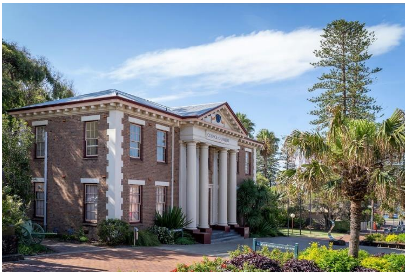
Figure 4: Kiama Council Chambers.
