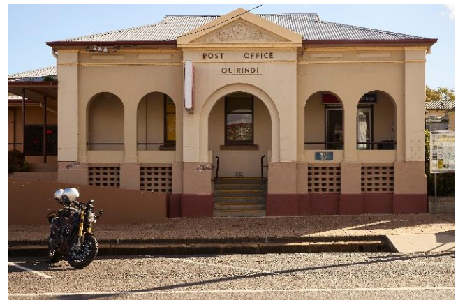
Figure 2: The historic Quirindi Post Office. Photo credit: Destination NSW.
