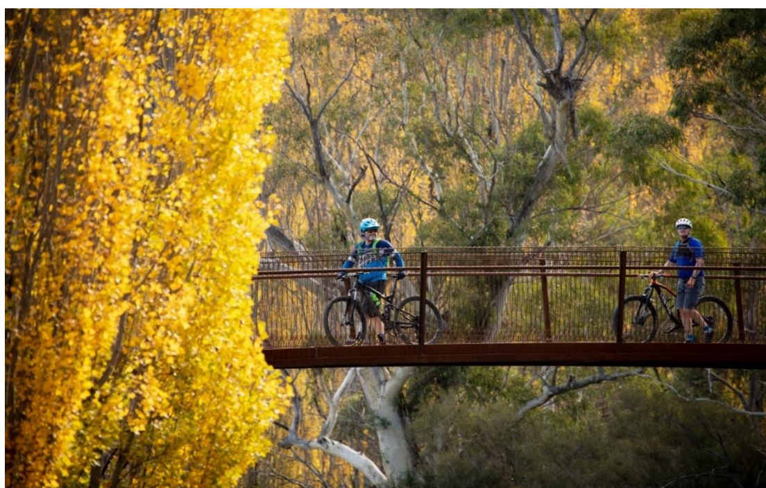
Figure 7: Lower Thredbo Valley Trail Bridge. Photo credit: Matt DeWard.
