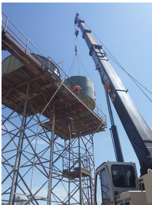
Figure 19: Water bores at Pooncarie in Wentworth LGA. Photo credit: Wentworth Shire Council.
