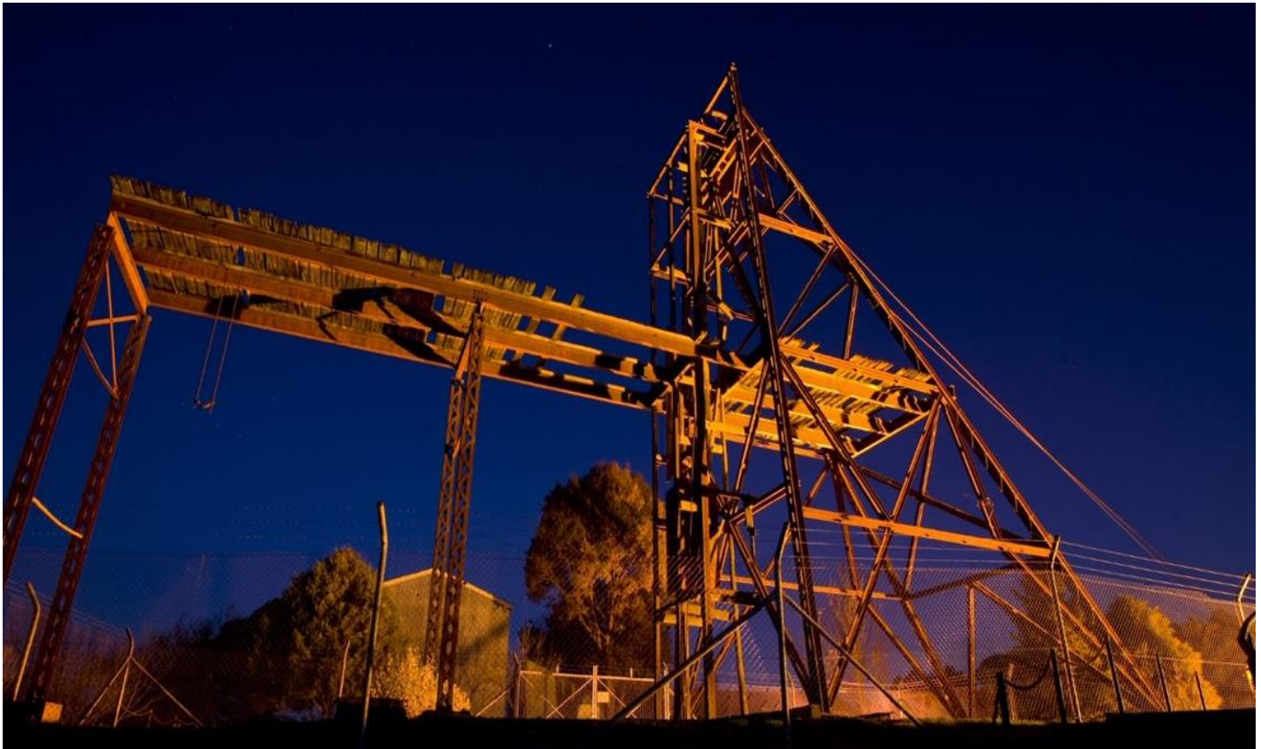
Figure 7: Wentworth Mine, Lucknow. Photo Credit: Orange City Council.
