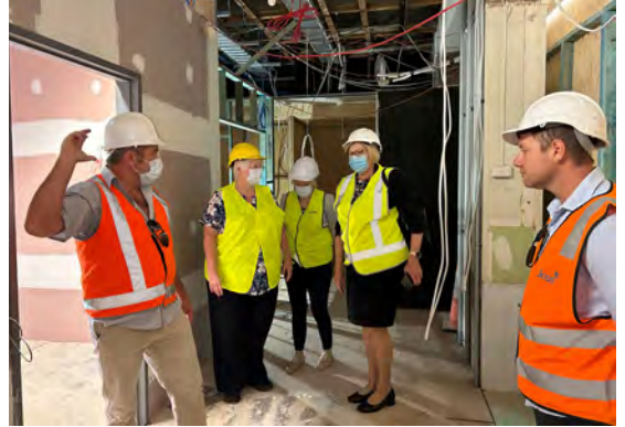
Construction progress at Leeton Hospital Emergency Department
